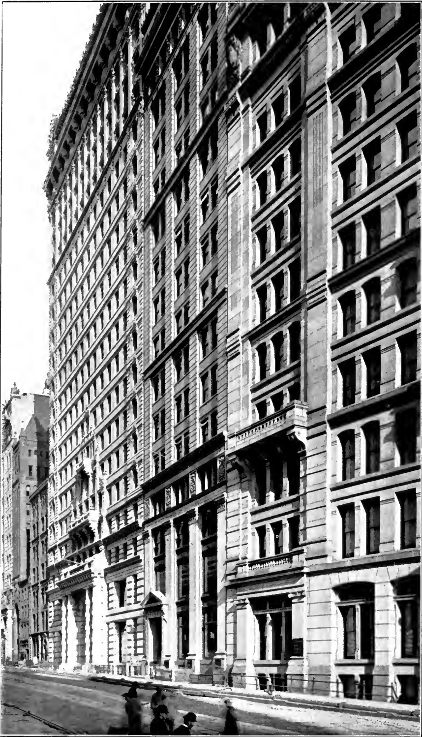
FIG. 2. NOS. 26-42 BROADWAY—THE FRONT.
